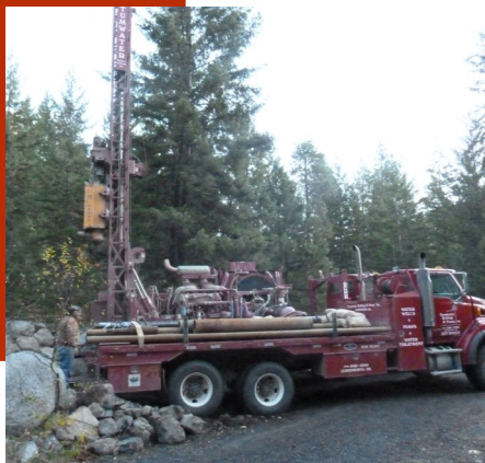
The Well Drilling Rig on site at Ingalls Creek
